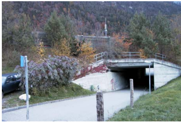
Fig. 5b Concrete underpass
