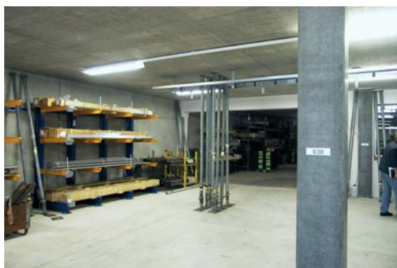
Fig. 10c Test with eight struts in midspan to achieve an increase from 14 Hz to 18 Hz
