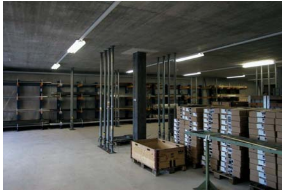
Fig. 10a Test with eight struts near each column to achieve doubling of eigenfrequency
