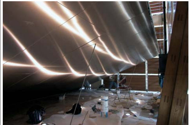
Fig. 9b Rear view; 2 tension cables between the free edge of the cantilever platform and the floor beneath stiffen the system.
