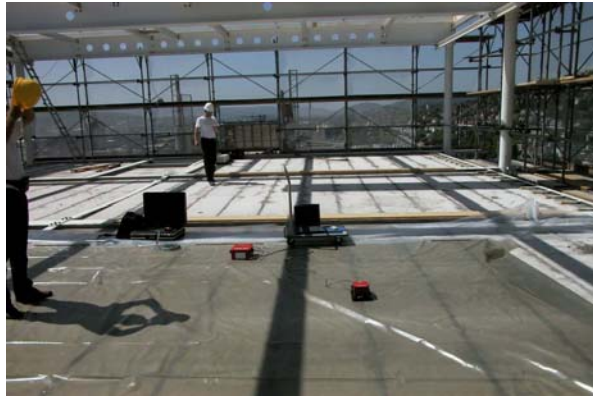
Fig. 8a Light-weight concrete floor slab in construction
