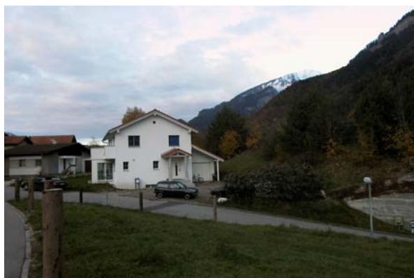
Fig. 5d Affected building
