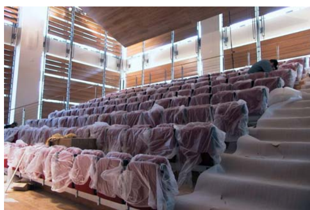
Fig. 9a Seat rows on cantilevered platform
