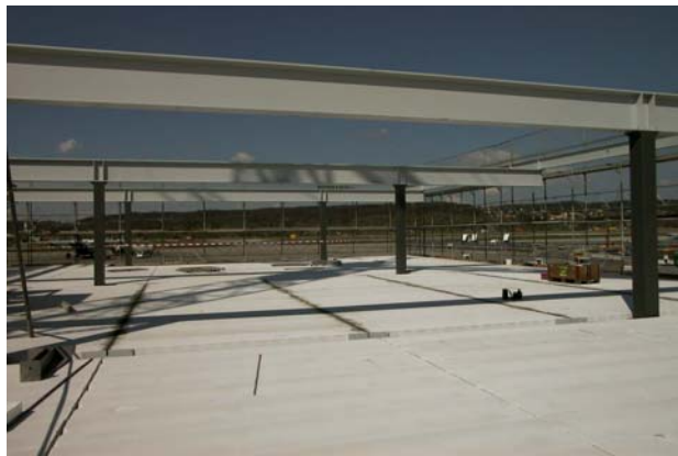
Fig. 7a Light-weight concrete floor slab for bus terminal
