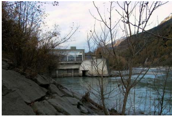
Fig. 5a Hydro power station
